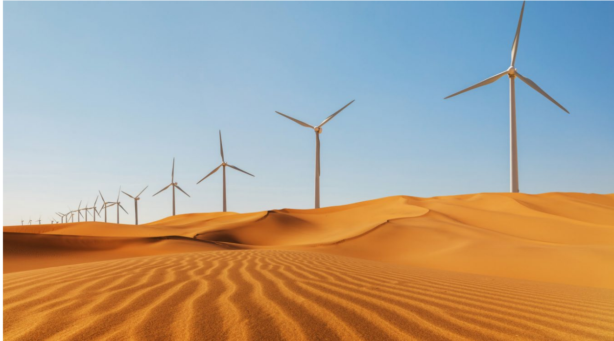
Wind turbines in the Sinai Desert, Hurghada, Egypt
