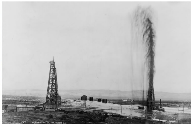
Left: Wooden derrick built ca. 1917 preserved at the West Kern Oil Museum in California. Photo by Konrad Summers (Wikimedia Commons, Creative Commons Attribution-Share Alike 2.0 Generic license, image resized and cropped) . Right: An oil field in California ca. 1910 with a gusher spewing oil on the right. Photo by West Coast Art Co. (from the Library of Congress Prints and
